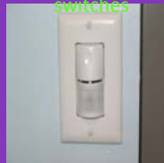
Motion sensitive light switches
